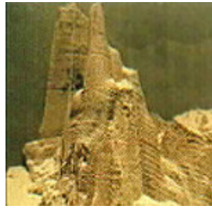
View of soya build up from down inside silo just prior to activation of one Cardox Tube.
