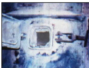
Before: Opening inspection holes reveals build-up of cement.
