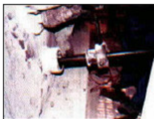
During: Cardox Tube is inserted into the build-up through special sockets.
